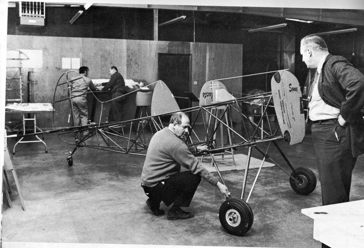
Airline captain, Sam Huntington watches Paul fit the rear landing gear tube. Sam later had the opportunity to fly the completed airplane. He stands 6' 5" and weighs 240 lbs.
